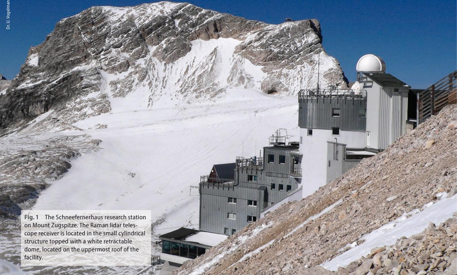
**Fig. 1** The Schneefernerhaus research station on Mount Zugspitze. The Raman lidar telescope receiver is located in the small cylindrical structure topped with a white retractable dome, located on the uppermost roof of the facility.
